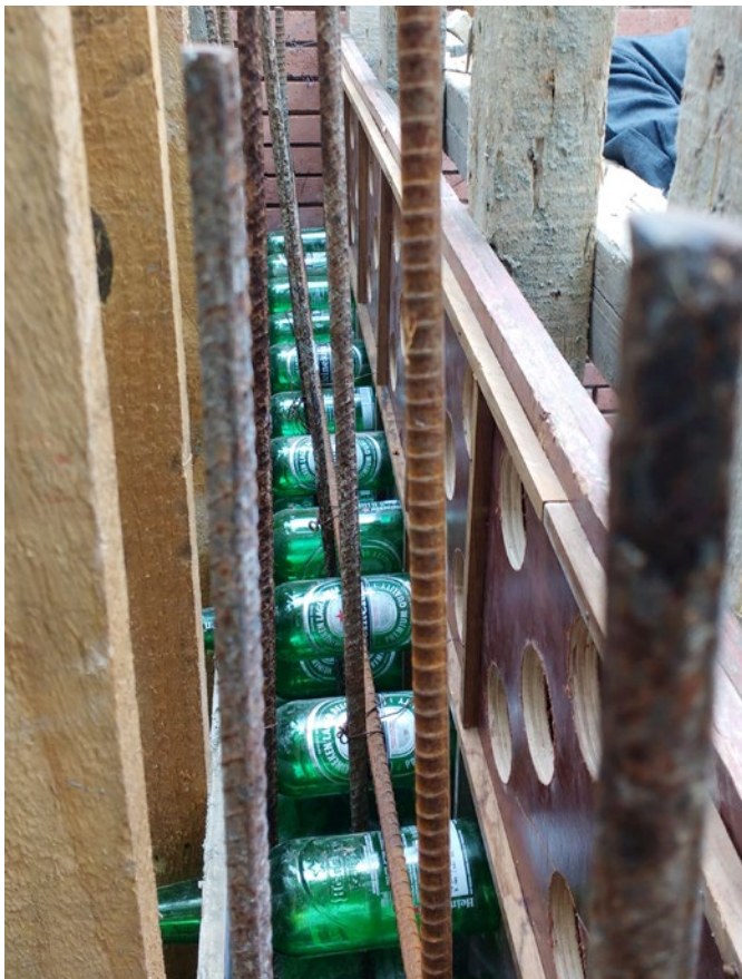
↑ Construction details of Filler Wall.
